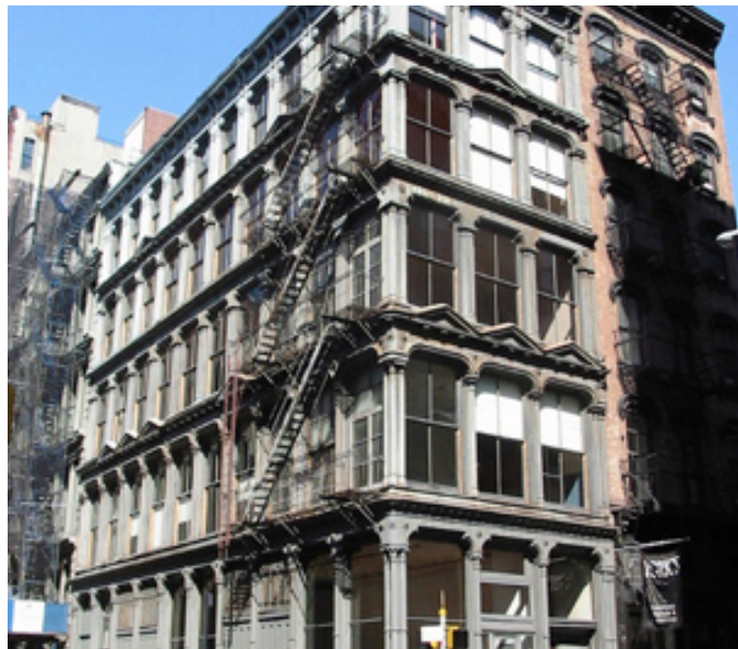
101 Spring Street, home of the Judd Foundation, is the only intact, single-use cast-iron building remaining in SoHo. Image courtesy of Judd Foundation Archive.
