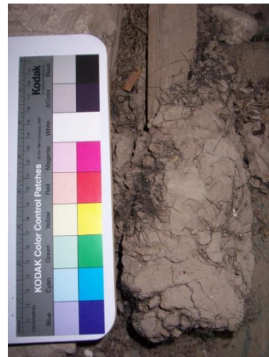
Figs. 8 & 9 (left): Loose bousillage at Parlange Plantation. Photographs by L. Blokker, 2008, with the funding support of an Old Salem Architectural Fellowship.
