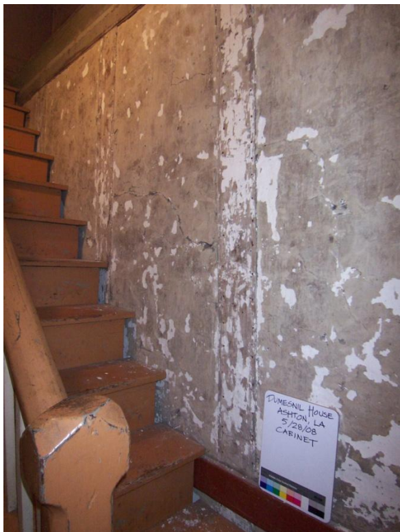
Figs. 10 & 11 (left and above): Interior bousillage wall at Dumesnil House and detail of cracked bousillage revealed by removal of chair rail. Photographs by L. Blokker, 2008, with the funding support of an Old Salem Architectural Fellowship.
