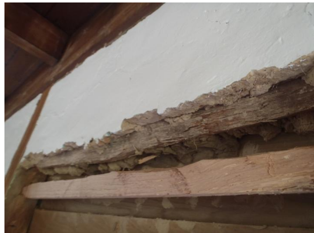
Fig. 5: Detail of original Hebert House bousillage and barreau above new barreau . Photograph by H. Knight.
