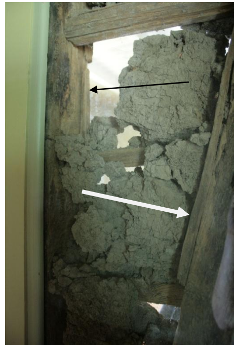
Fig. 4: Detail of bousillage with arrows indicating thin wood strips. Photograph by L. Blokker.
