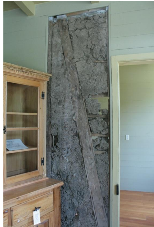
Fig. 2 (above): Preserved section of bousillage in Estopinal House. Fig. 3 (below): Close-up of bousillage section showing thin strips of wood affixed to brace, indicated by arrows. Photographs by L. Blokker.
