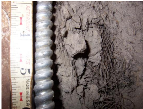
Figs. 12 & 13 (left): Bousillage in situ at the Desfossé House. Photographs by L. Blokker, 2008, with the funding support of an Old Salem Architectural Fellowship.
