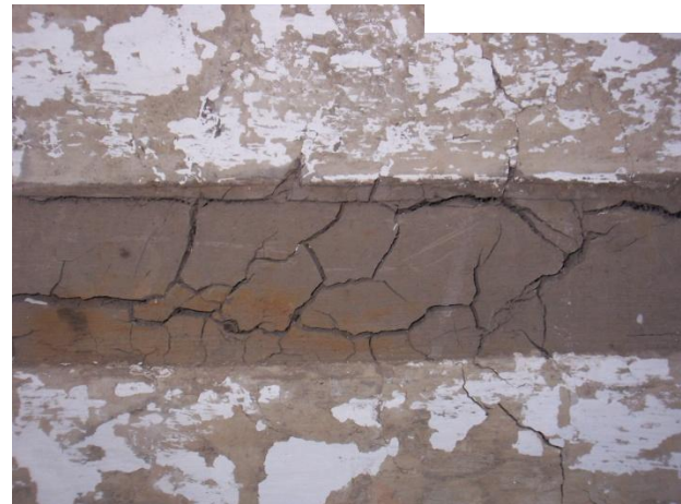
Figs. 10 & 11 (left and above): Interior bousillage wall at Dumesnil House and detail of cracked bousillage revealed by removal of chair rail. Photographs by L. Blokker, 2008, with the funding support of an Old Salem Architectural Fellowship.
