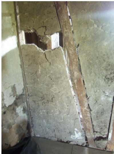
Figs. 14 & 15 (right): Bousillage in situ at Mather House. Photographs by L. Blokker, 2008, with the funding support of an Old Salem Architectural Fellowship.
