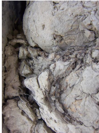
Figs. 6 & 7 (left): Bousillage in situ at Homeplace Plantation. Photographs by L. Blokker, 2008, with the funding support of an Old Salem Architectural Fellowship.
