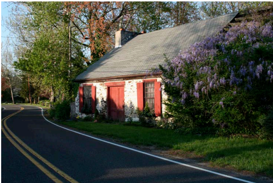
A very narrow clear zone in the New Jersey Pinelands. Paul Daniel Marriott
