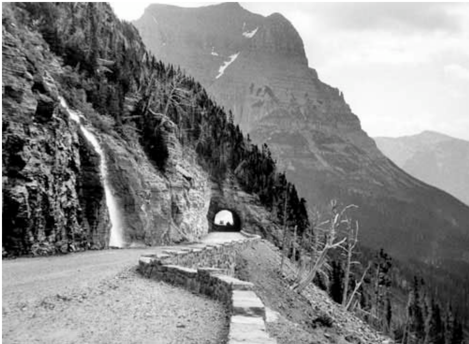
The Going-to-the-Sun Road at Glacier National Park, Montana, was the first automobile road in a National Park. 1933 image with macadam (crushed stone) pavement. National Park Service
