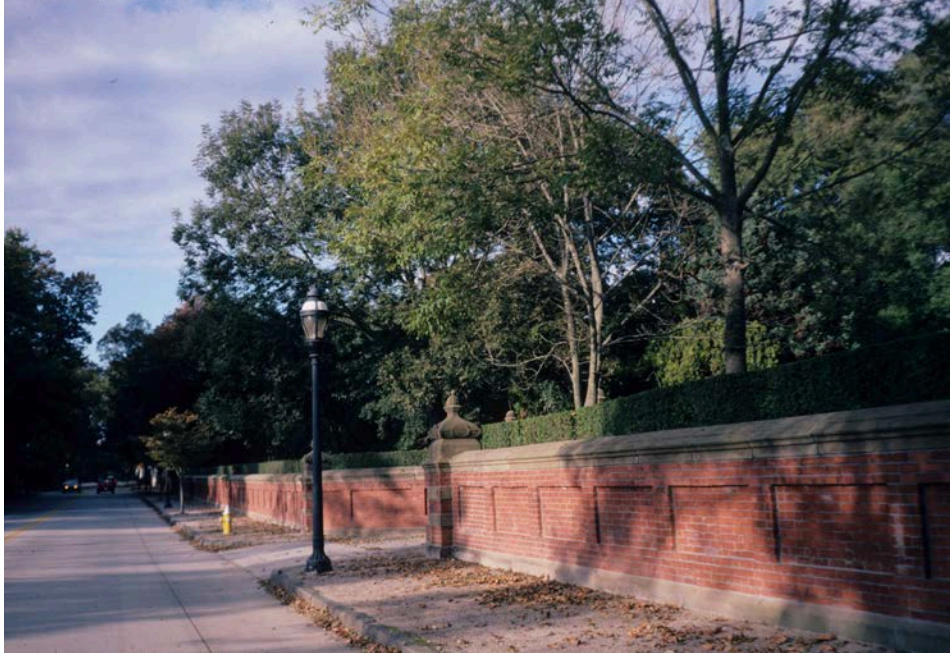
Bellevue Avenue in Newport, Rhode Island was determined to be beyond repair in the 1980s. As a contributing element to the Bellevue Avenue National Landmark District (1976), the Rhode Island Department of Transportation reconstructed Bellevue Avenue in 1991 using the original 1924 concrete specifications. The historic gravel sidewalks were made ADA compliant by the addition of an asphalt subsurface for improved stability. Paul Daniel Marriott
