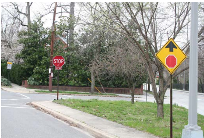
There is a growing tendency to over-sign as seen here with an “Advance Traffic Control” (stop ahead) sign in Washington, DC. This sign violates MUCTD guidance that states: “These signs should be installed on an approach to a primary traffic control device (the stop sign, in this illustration) that is not visible for a significant distance.... ” (MUTCD Section 2C.29, emphasis added). MUTCD further recommends that advance traffic control signs on posted 25 MPH streets—as in this illustration—should be located 350 in advance if the stop sign is “not visible.” This sign is approximately 40 feet from the stop sign. Paul Daniel Marriott
