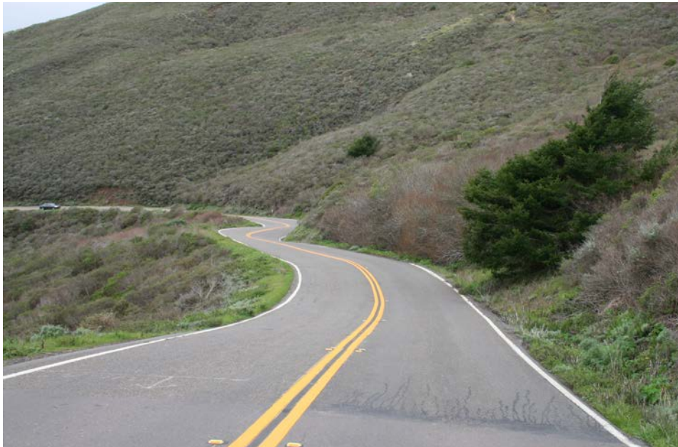
Horizontal alignment (curves) on California Route 1 in Marin County. Paul Daniel Marriott
