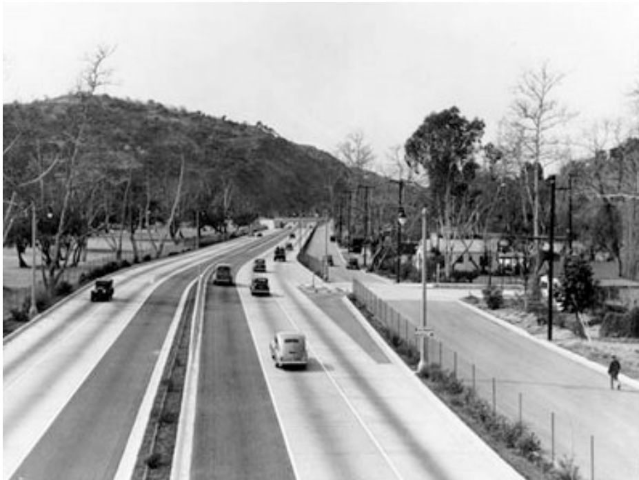
The Arroyo Seco Parkway, between downtown Los Angeles and Pasadena, California, opened in 1940. It combined both parkway qualities and emerging freeway concepts. Highland Park Heritage Trust
